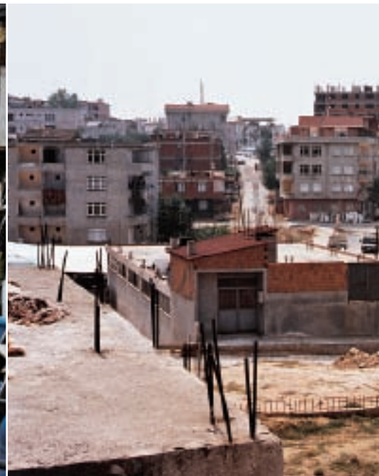
Squatters' homes near Istanbul, Turkey; the rebar allows for expansion
